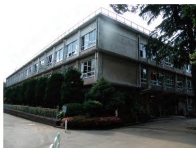
附属中学校第Ⅰ校舎 Junior High School Building I
