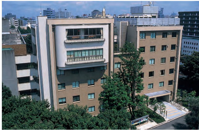
理学部 3 号館 Faculty of Science, Building 3
