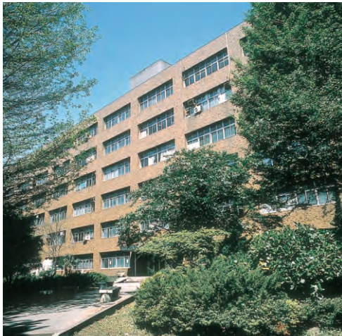
理学部 1 号館 Faculty of Science, Building 1
