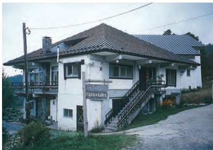
志賀高原体育運動場 Shiga Heights Physical Training Facility
