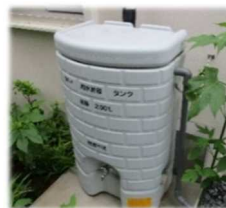
Rainwater storage tank
