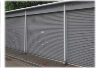
Industrial waste storage
